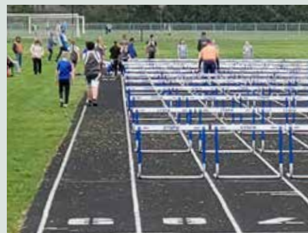
Top: The well-used worn out track at CTSFW
